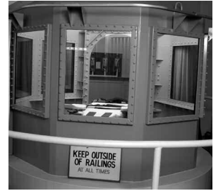
New San Quentin execution chamber.
